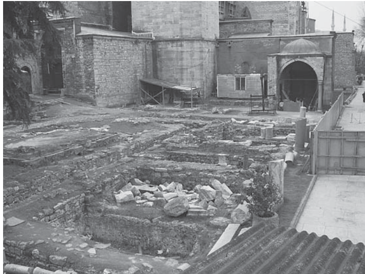
Fig.11 Even areas off-limits to the public must be kept tidy and orderly.
