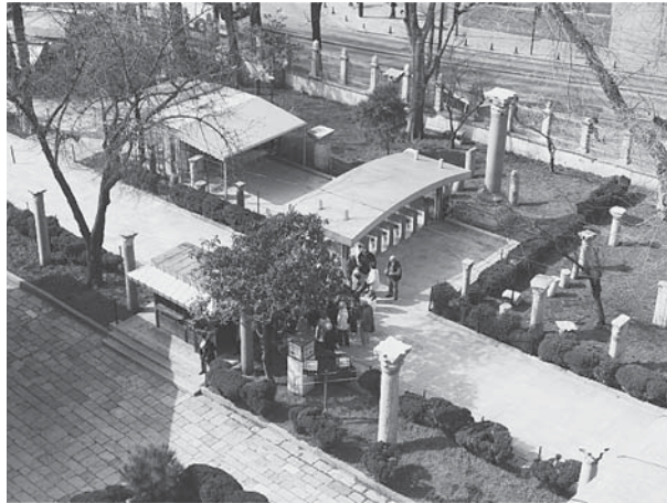
Fig.14 Entrance security gate
