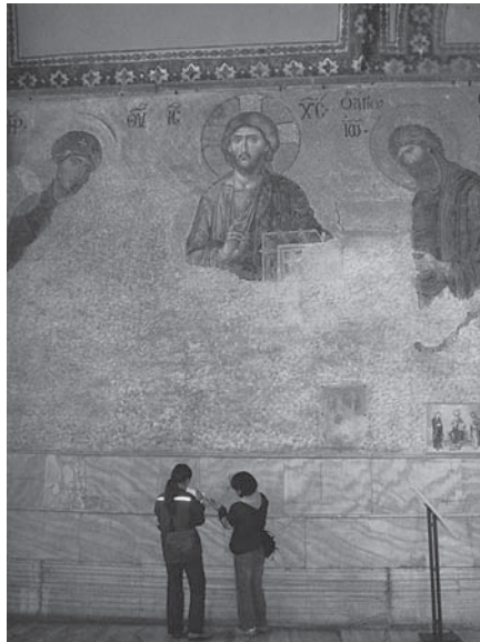
Fig.5 Survey of extent of peeling of mosaics
